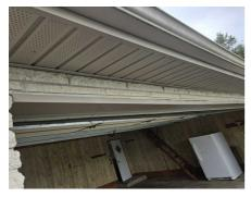
• Metal wrapping around vehicle door jamb loose at top, suggest securing and sealing.
