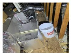
• Attempts made to protect condensation lines from freezing, suggest corrections by qualified specialist that may include use of heat tape
