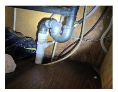
• Improper wasteine hook up after the trap under the sink, suggest corrections to connect prior to the trap.
