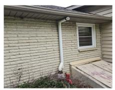
Notes: Terminates improperly, potential for gases to be drawn back in window
