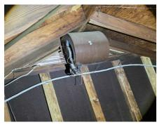
• Rigged vent/ blower installed at left end, not wired, suggest removal
