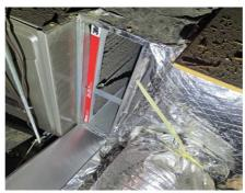
• Dirty Air Filter Observed. Furnace filters should be changed every three months. Dirty filters can lead to costly system repairs, as well as allow dust buildup, animal dander, pollen and other unwanted allergens into a homes air system. It is suggested to have a qualified specialist make repairs as needed.
