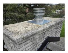
• Crown does not have a fully built up mortar bed to shed water out and away, suggest monitoring and maintain seals and joints or preventative crown build up.
