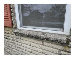
• Window weep holes blocked at left side garage, suggest corrections so water does not get trapped.
